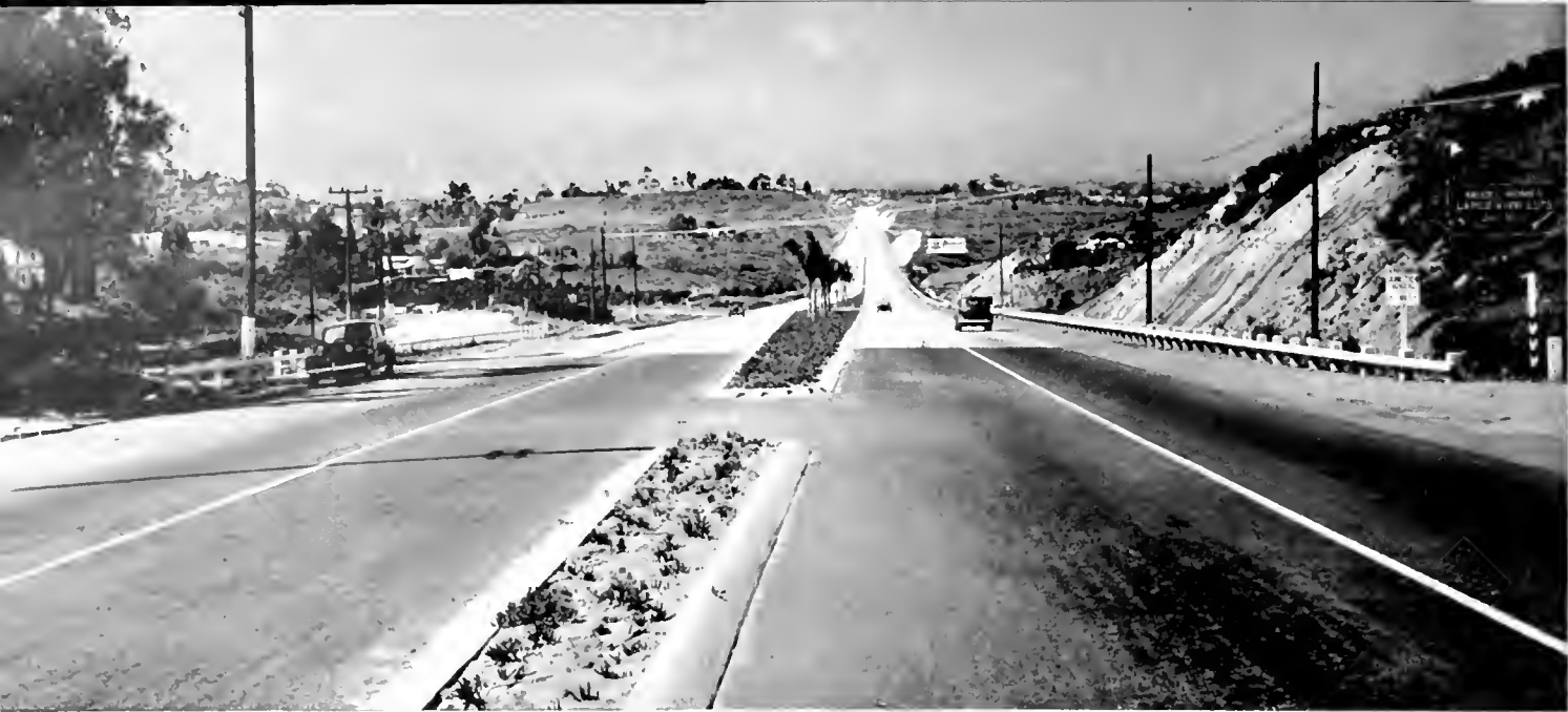
This section of four-lane divided highway of modern design is paved with both asphaltic concrete and portland cement concrete
